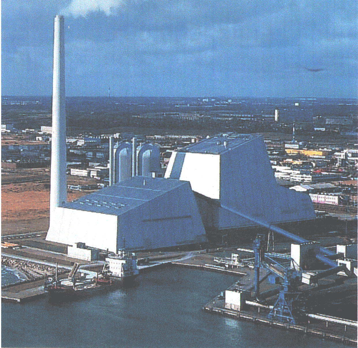
Avedøre Power Station 1. Fired with coal and fuel oil. Courtesy Avedøre Power Station.
