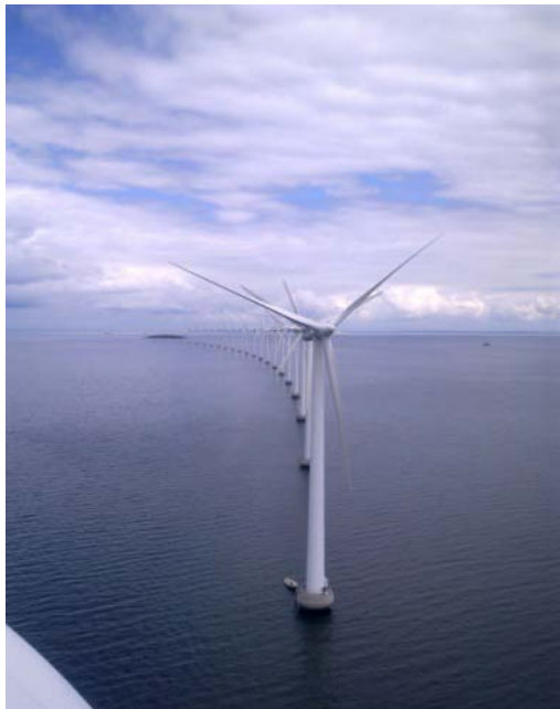
Figure 3-4. Middelgrunden Wind Plant (HC Sorensen, Middelgrunden Wind Turbine Cooperative, NREL/Pix 17855)
