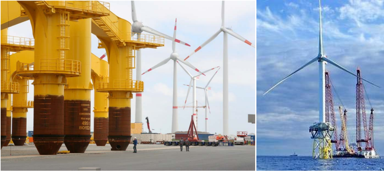
Figure 5-8. Transitional substructure technology under development: BARD 1 foundation structures awaiting loadout with 5-MW AREVA and REpower test turbines in background (Gary Norton, DOE NREL/PIX 17889); submerged four-pile jacket with transition to tube tower on Talisman Energy project with REpower 5-MW turbine (right, Talisman Energy, NREL/PIX 17885) (MacAskill 2005)
